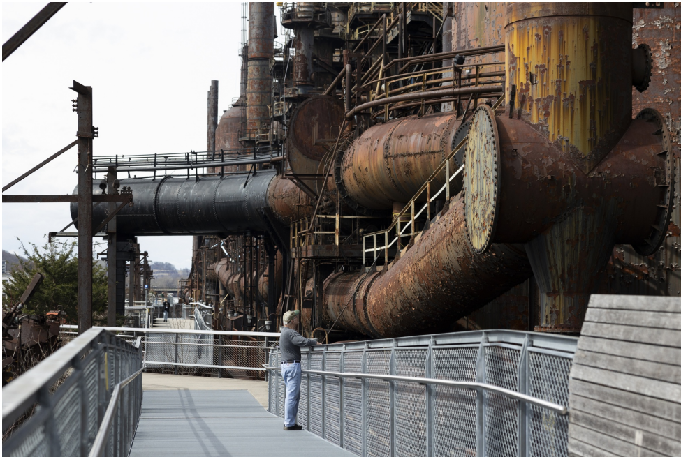
A pedestrian bridge allows visitors to get a closer look at the Bethlehem Steel Stacks in Bethlehem.
